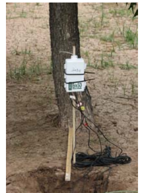
Example of a soil moisture sensor installed in the field
