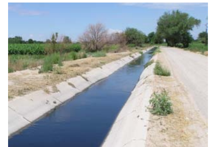
Aguas negras or "black water" wastewater canal, Juarez Valley, Mexico
