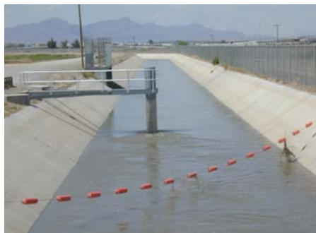
Lined American Canal Extension in El Paso
