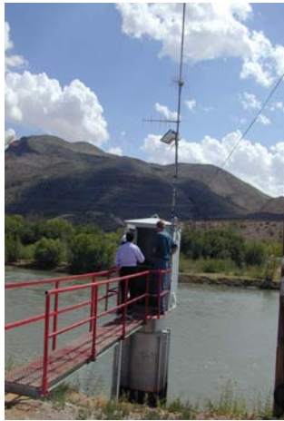
Telemetry Gage Station
